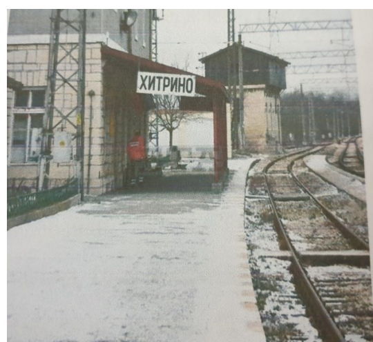
Figure 10. The train station in the village of Hitрино before the explosion on 10.12.2016.
